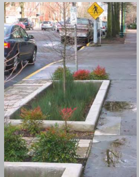
Street runoff collects in stormwater planters in Portland, Oregon.
