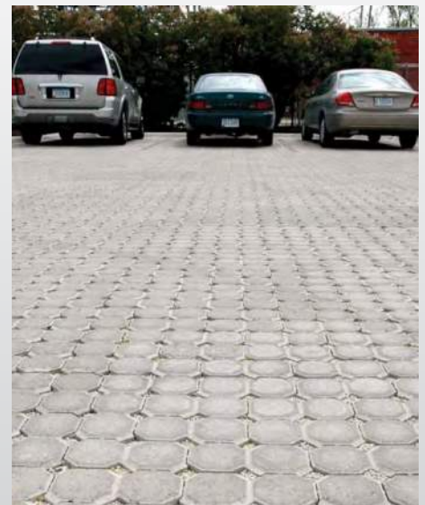
Rainfall soaks through permeable pavement and into the ground below in this parking area in west Des Moines, Iowa.
