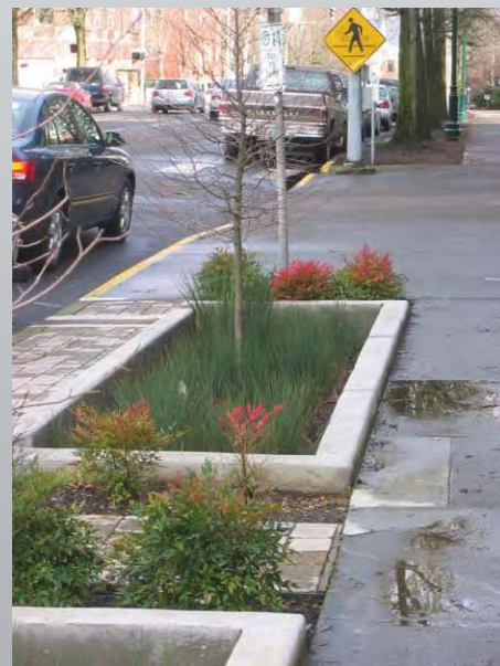
Street runoff collects in stormwater planters in Portland, Oregon.
